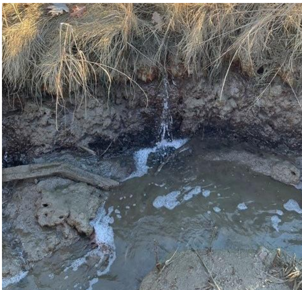
Discharge from subterranean ditch voids indicates clay-cored embankment use at Smelt Brook Preserve
