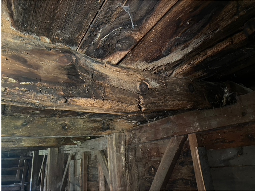
A rotted floor joist beam on the verge of collapse.
