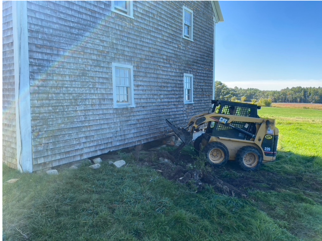
Removing the unstable foundation stones.
