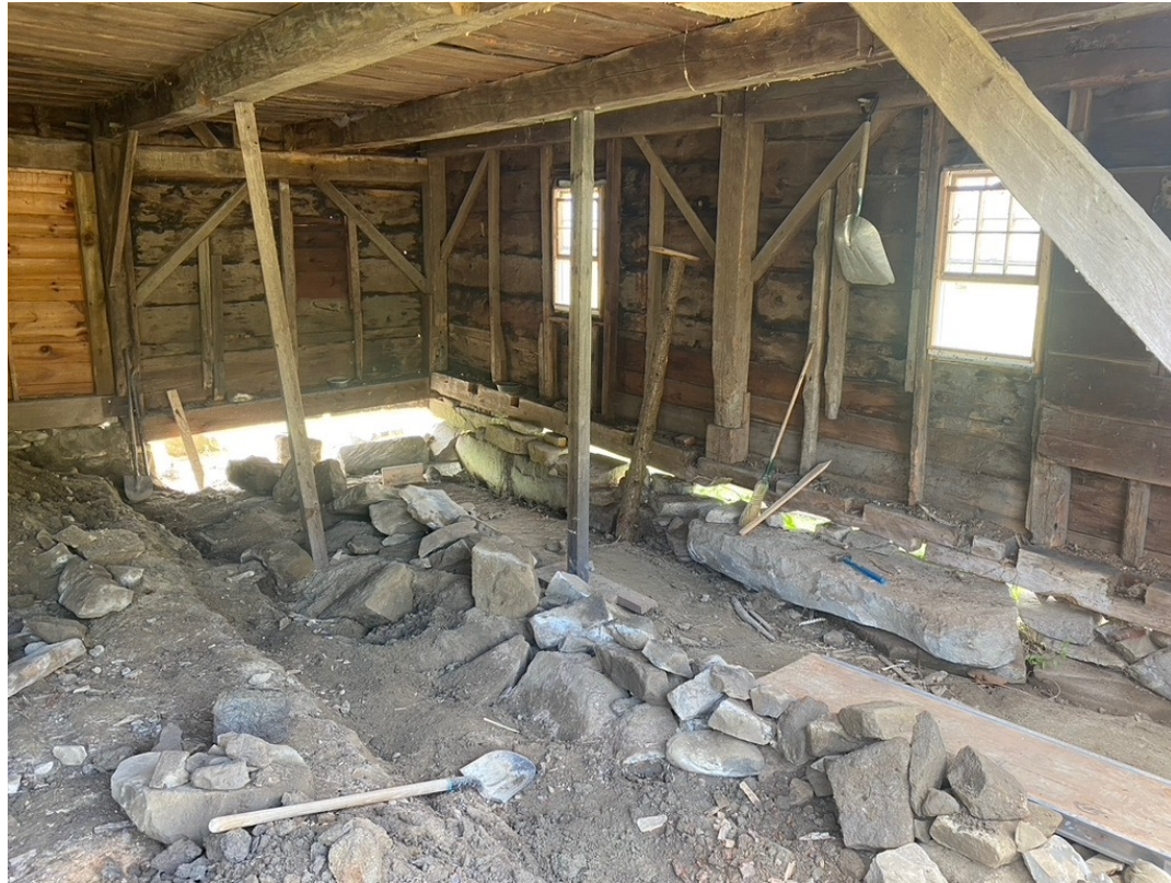
The north wall had shifted outward off the foundation.
