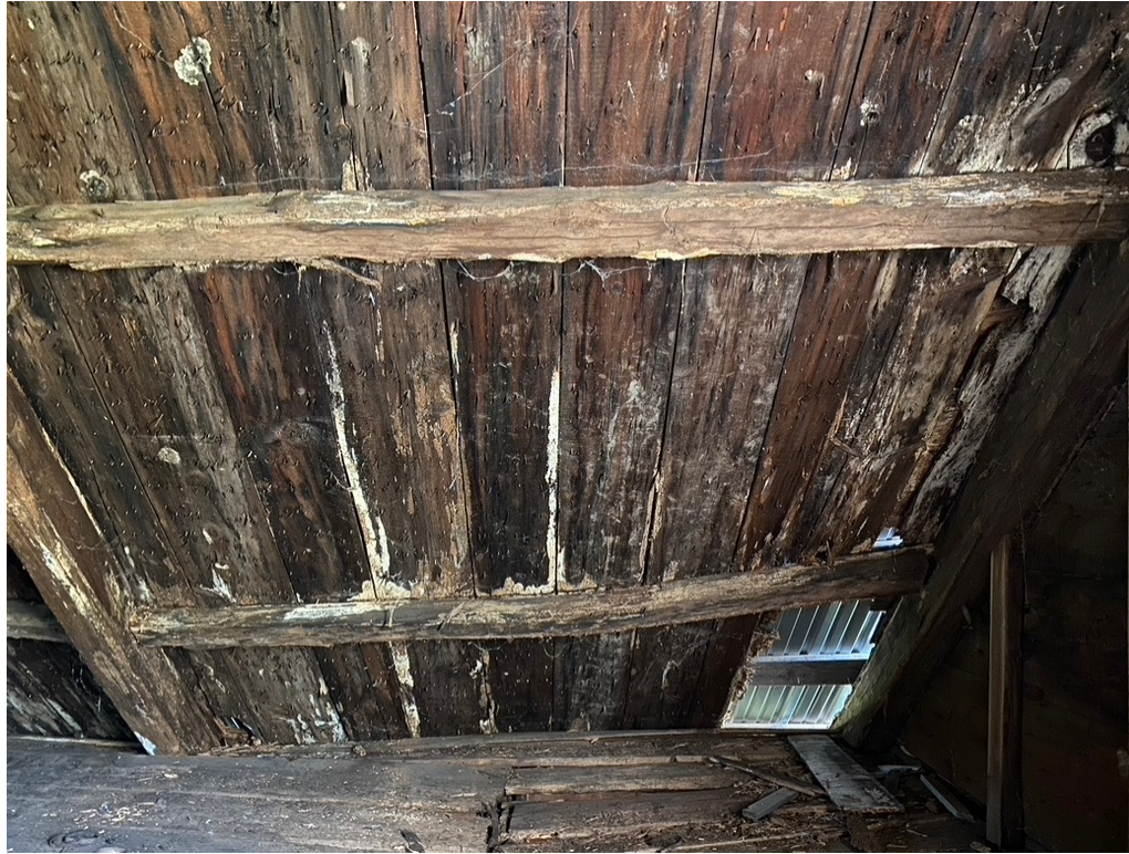
Compromised roof boards due to water infiltration.
