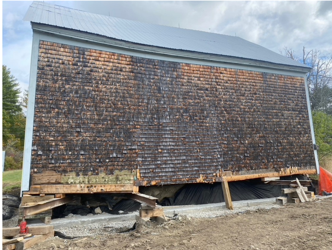
The completed west side concrete footing.
