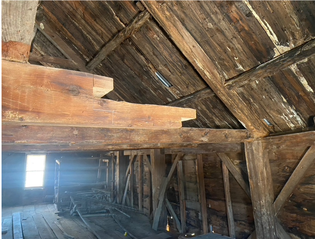
The collapsing floor joist beam with rotted wood removed, ready for splicing in 2026.
