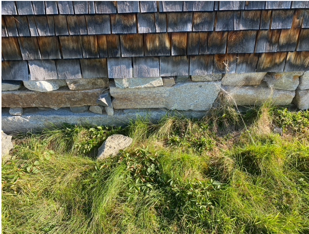
An unstable foundation with repurposed cemetery stone posts.
