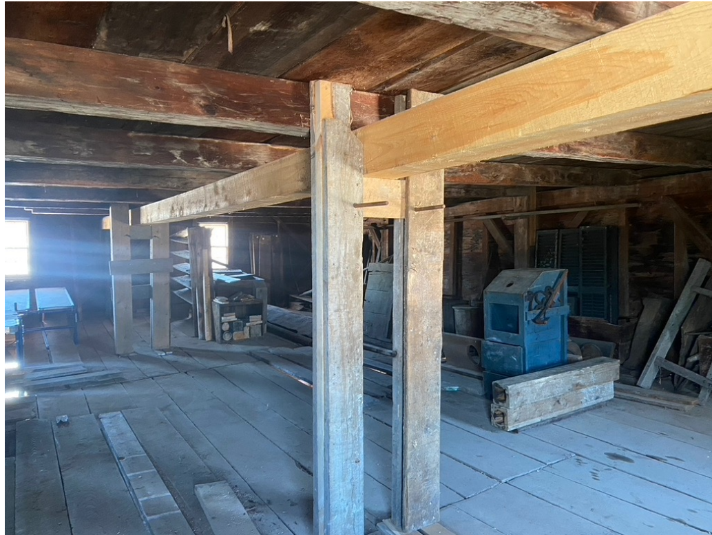
The 40-foot hemlock support beam on the second floor. A matching beam was installed on the first floor.
