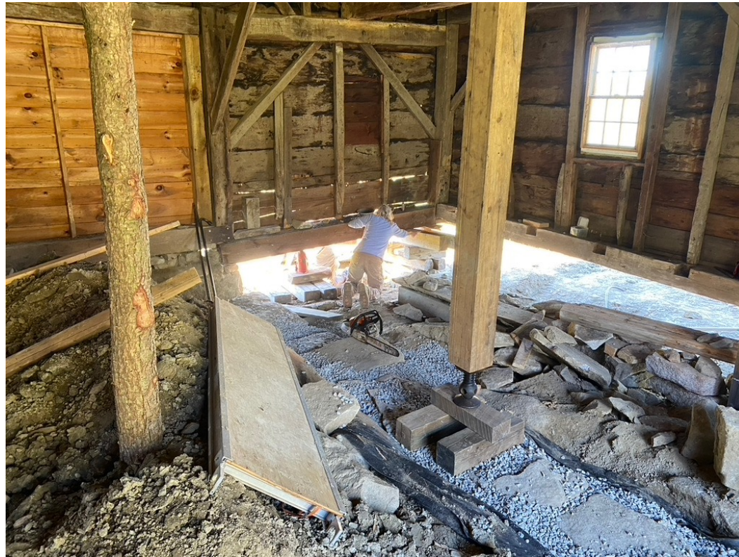
Preparing to dig foundation trench.
